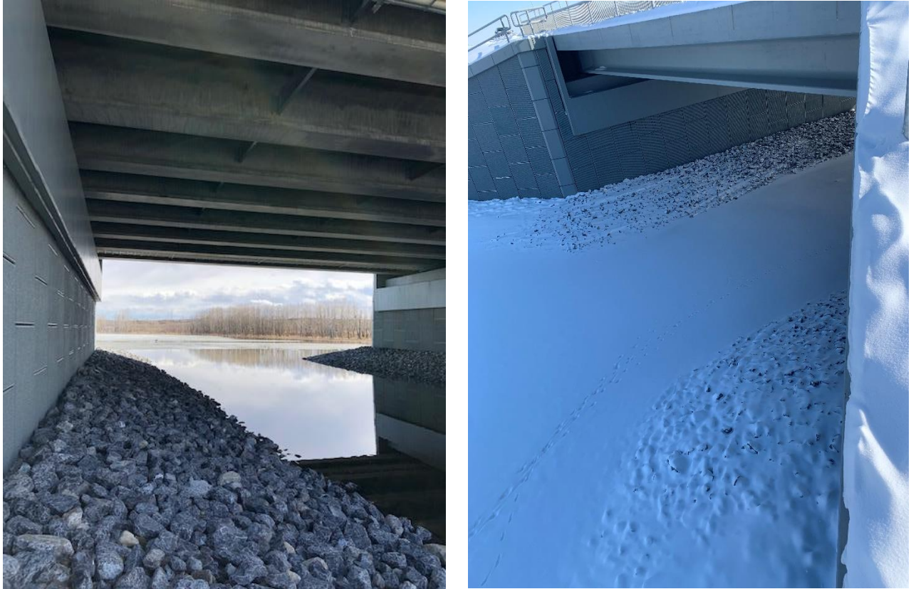
Figure 10: Photos of the underpass substrate and surface during summer (left panel—deer attempted but were not able to cross) and winter (right panel—deer successfully crossed).
